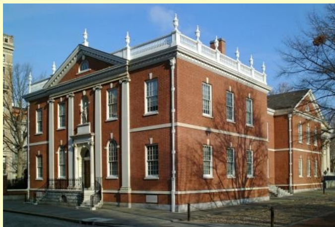
Library Hall from 5th Street
